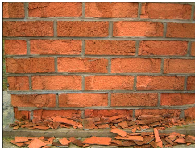
Figure 3.1. Frost damage to brick masonry (Smith & Edgell 2009, p.4).
