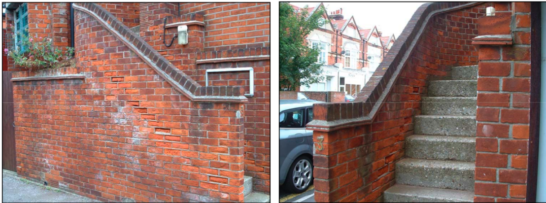
Figures 3.13 and 3.14. Localised frost damage in bricks. Pooling water on the stair treads has caused increased saturation on freezing (Smith & Edgell 2009, p.5).
